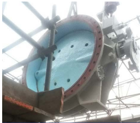
Refurbished 72" butterfly valve
