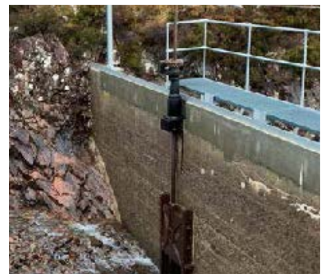
Penstock supply and installation
