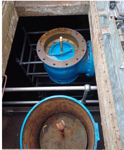
The Refurbished Valve before the installation of the cover and the lever arm
