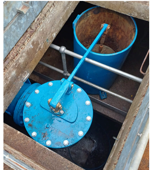
The Refurbished Valve Reinstalled Within the Service Reservoir
