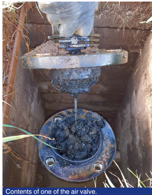
Internal float of the air valve with build up
