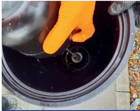
Cleaned internal of one air valve
