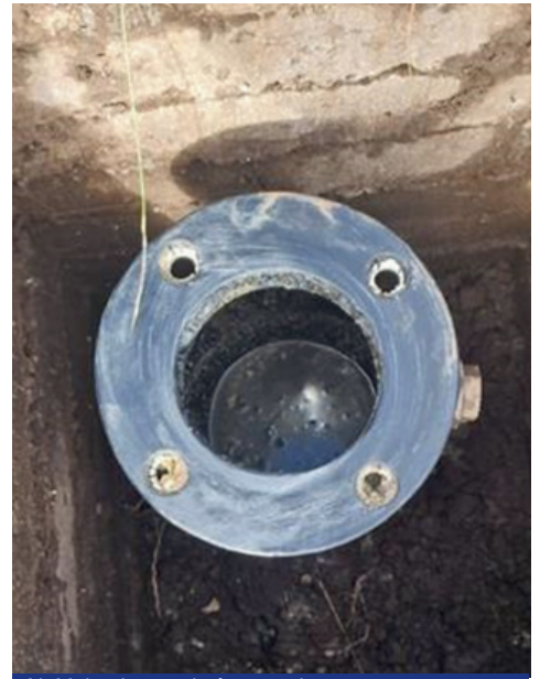
Air Valve internal after service
