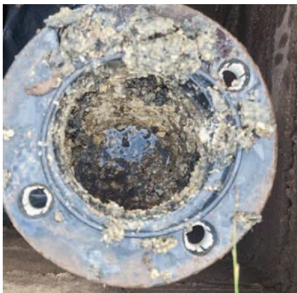
Build up of grease, making the air valve inoperable
