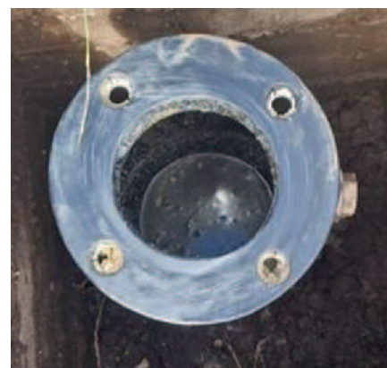
Air valve Internal after service
