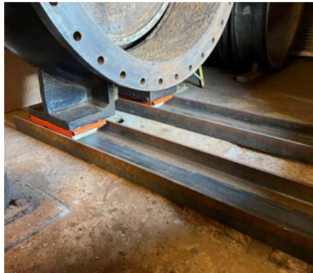
Skates used to move valves
