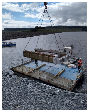
Bulkhead being loaded onto Pontoon.
