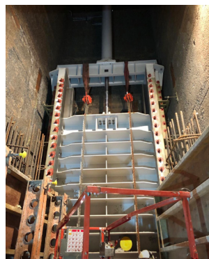
Secondary Scour Gate in position.
