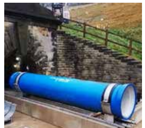
Section of new 900mm ductile pipe
