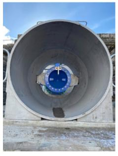
The outlet cone ensures that discharge is in the form of a hollow expanding jet, which is ideal for energy dissipation as the water is spread over a rapidly increasing surface area, thus permitting effective atmospheric cushioning. If partial /controlled containment of the jet is desired (such as for Burnhope Reservoir), a hood can be installed downstream of the valve.
