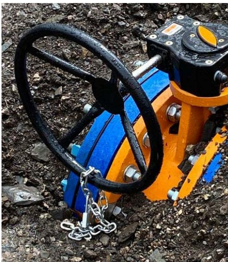
Locking of hand-wheel for security
