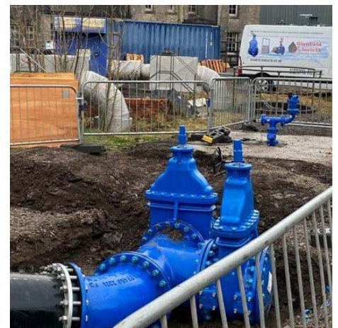
Installation prior to backfill
