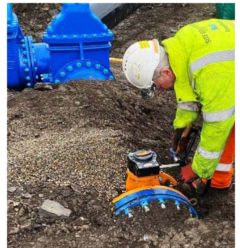
Setting of valve open position
