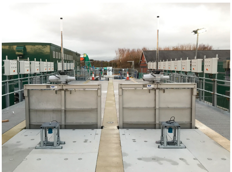
Penstock undergoing factory leakage and function testing.
